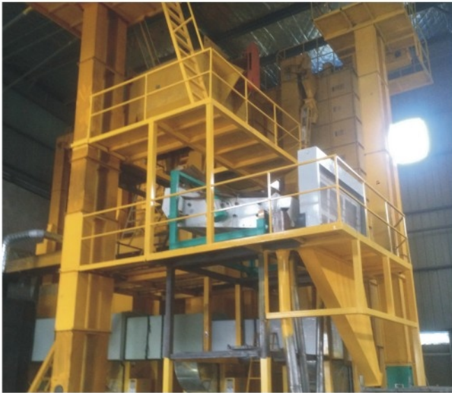
工程改造后 After The Engineering
