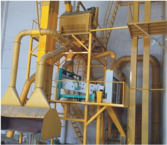
工程改造后 After The Engineering
